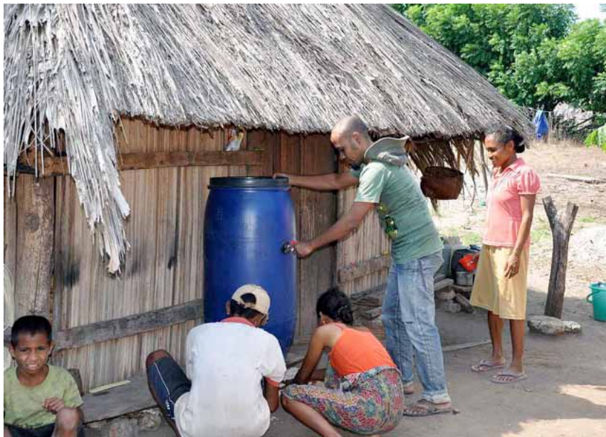
Installation of a bio-sand filtration unit.
