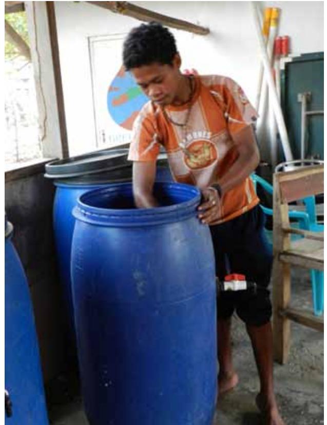
Building a Bio-sand filtration unit.
